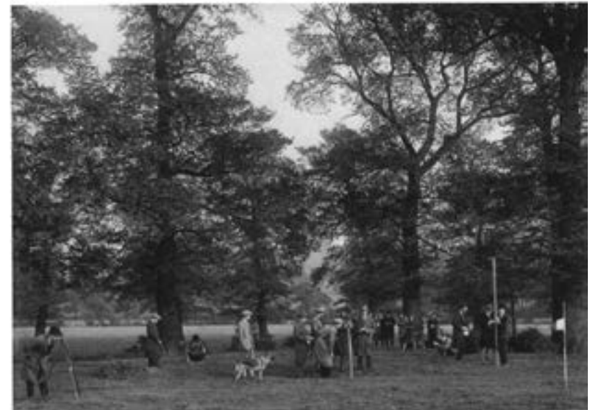
Clearing the land in 1903
